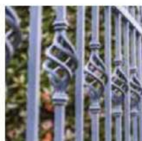
RAILING MS RAILING WITH ENAMEL PAINT FINISH
